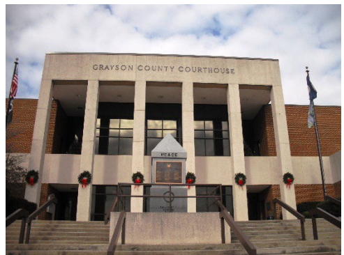
Figure 1-3: Grayson County Courthouse -Today
