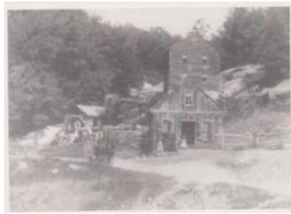
Figure 2-4: Powerhouse falls circa 1880s, Photo courtesy of the Grayson County Historical Society
