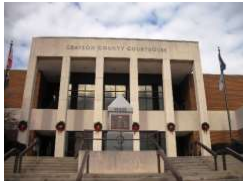
Figure 1-3: Grayson County Courthouse -Today
